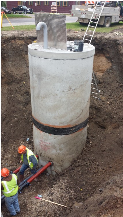
Lift Station Wet Well
