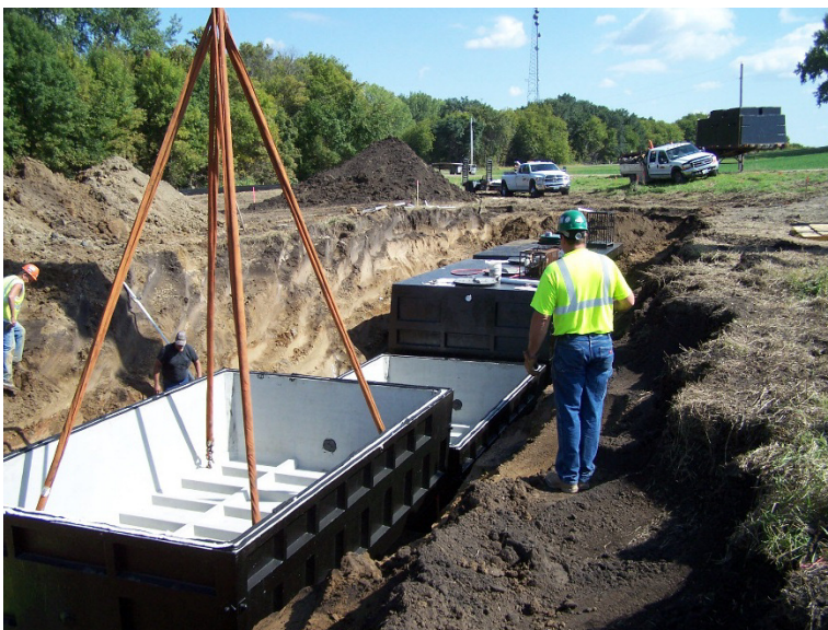
Four(4) 12,000 gallon Septic Tanks in Series
