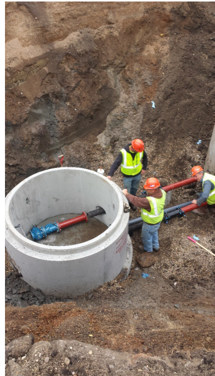
Lift Station Valve Vault
