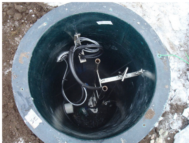
Residential Grinder Pump Station
