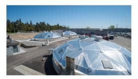
50 feet in diameter and has 16 feet side water depth. During the current upgrades, each clarifier was provided with new dome covers and drive motors were also upgraded to meet electrical code requirements. The domes reduce freezing issues during low flow winter months.
