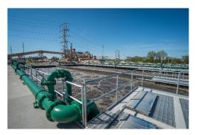
3.94 million gallons (MG). Each basin has fine bubble diffusers and air is supplied by four blowers. The blower system consists of one high efficiency hybrid blower and three high efficiency turbo blowers. A combination of these blowers is used to meet the
