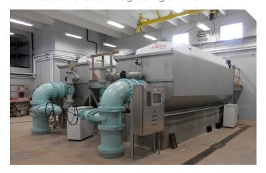
Design and Bidding of the new Tertiary Filter Building was completed by the end of 2015, with construction beginning in May 2016. The project is currently operational and substantially complete. The new treatment facilities will provide an economical, high quality effluent, meeting strict effluent standards for years to come and contribute to better water quality in the East Swan River Watershed and the Lake Superior Basin.
